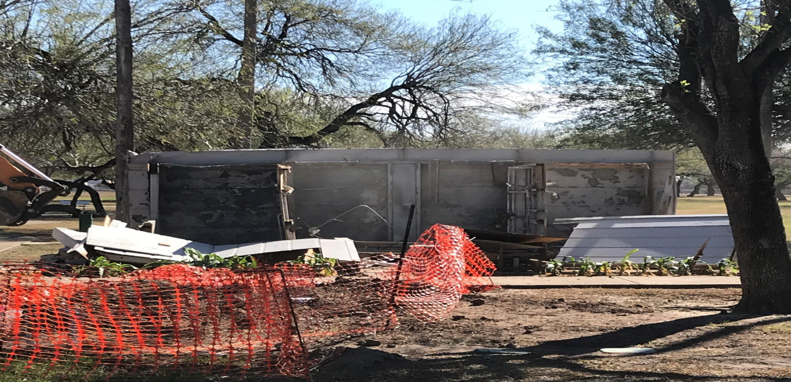
AIRPORT PARK EXISTING RESTROOM DEMOLITION
