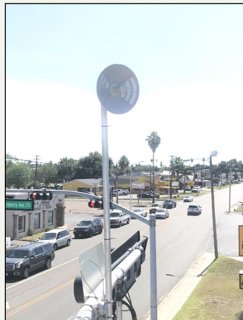
Upgraded Cabinet & Internal Hardware (Left) and Installation of Wi-Fi Antenna (Right)
