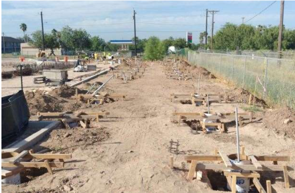
Magic Tunnel Footing
