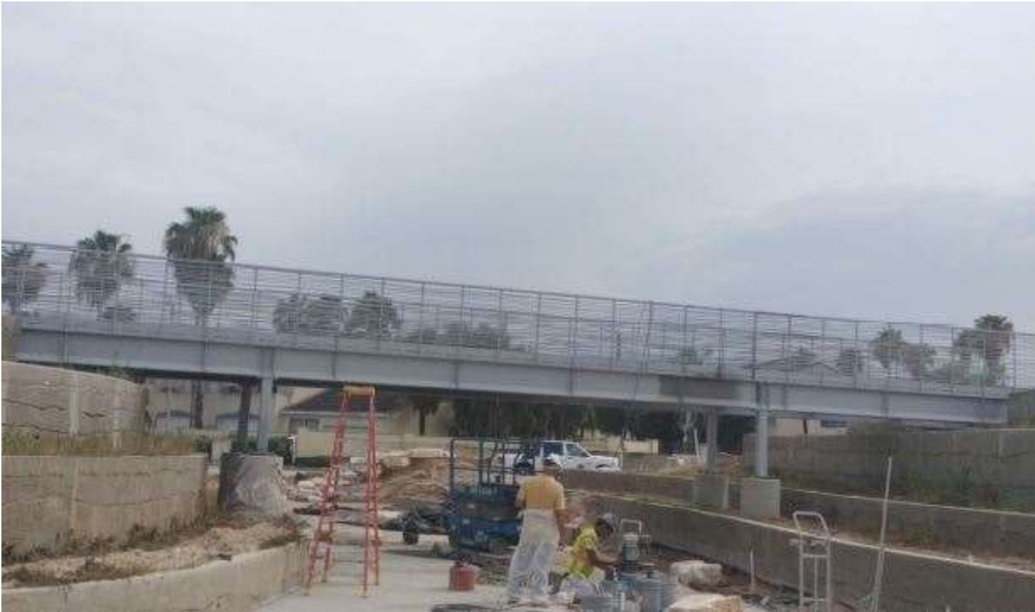
Rio Gorge Bridge
