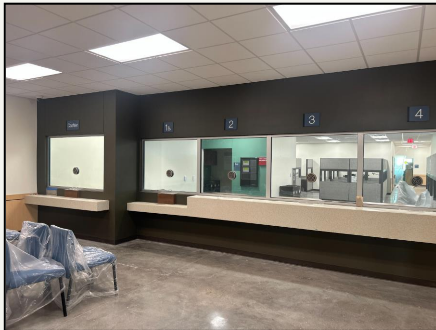
Outbound Administration Building Reception Area
