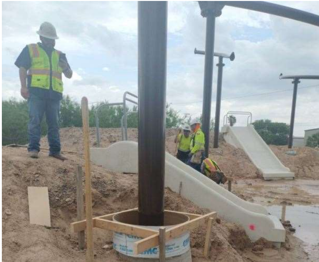
Embankment Concrete Slides
