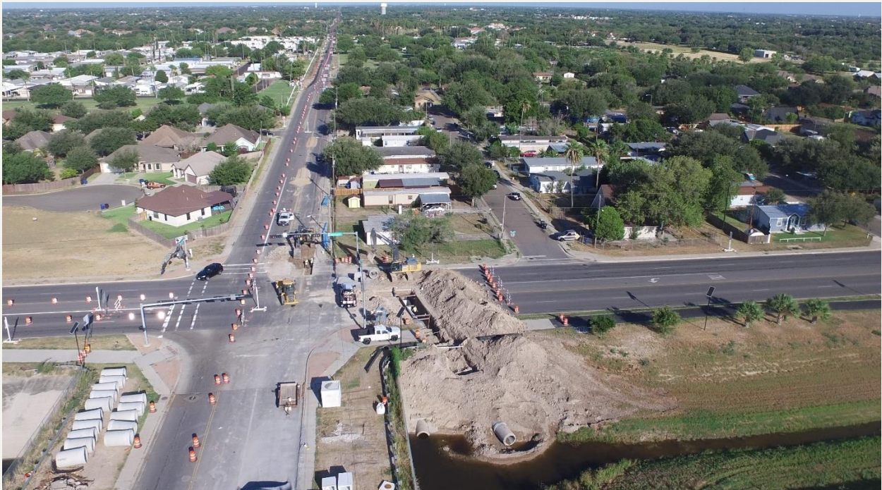
Figure 1. Installation of Daffodil Avenue Storm Sewer Infrastructure at Mission/McAllen Lateral
