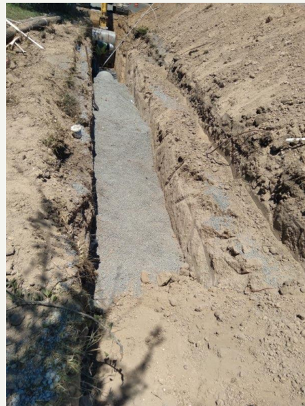
Storm Sewer installation
