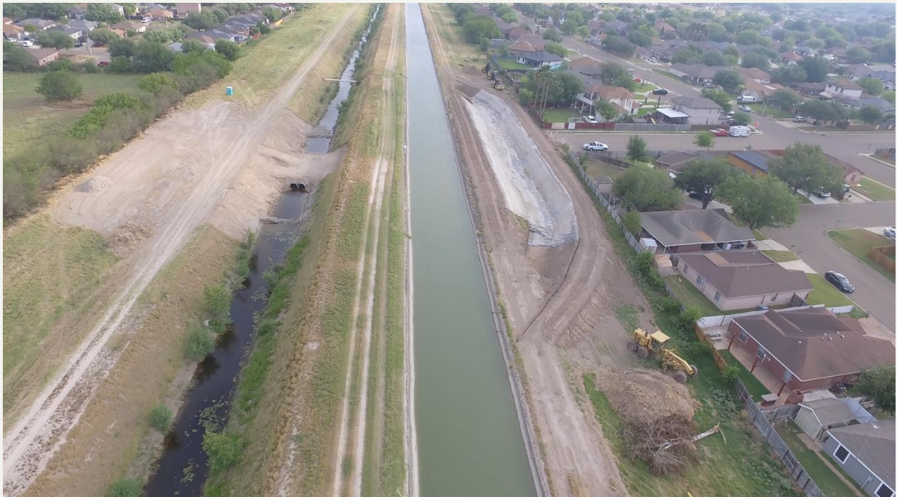
HCIDN1 Irrigation canal by-pass for construction of siphon crossing.
