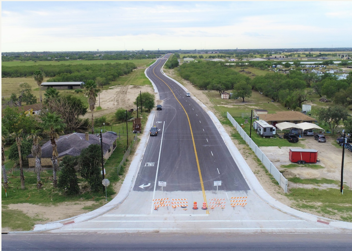
Freddy Gonzalez Dr. – Completion pending construction of HCWID No.1 infrastructure, replacement of broken inlet tops and failed concrete sidewalk replacement.
