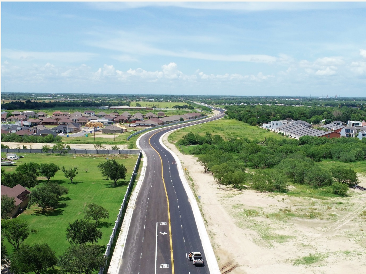
Bicentennial Blvd. Final Installation of Asphalt Surface Pavement at Freddy Gonzalez Drive Intersection.
