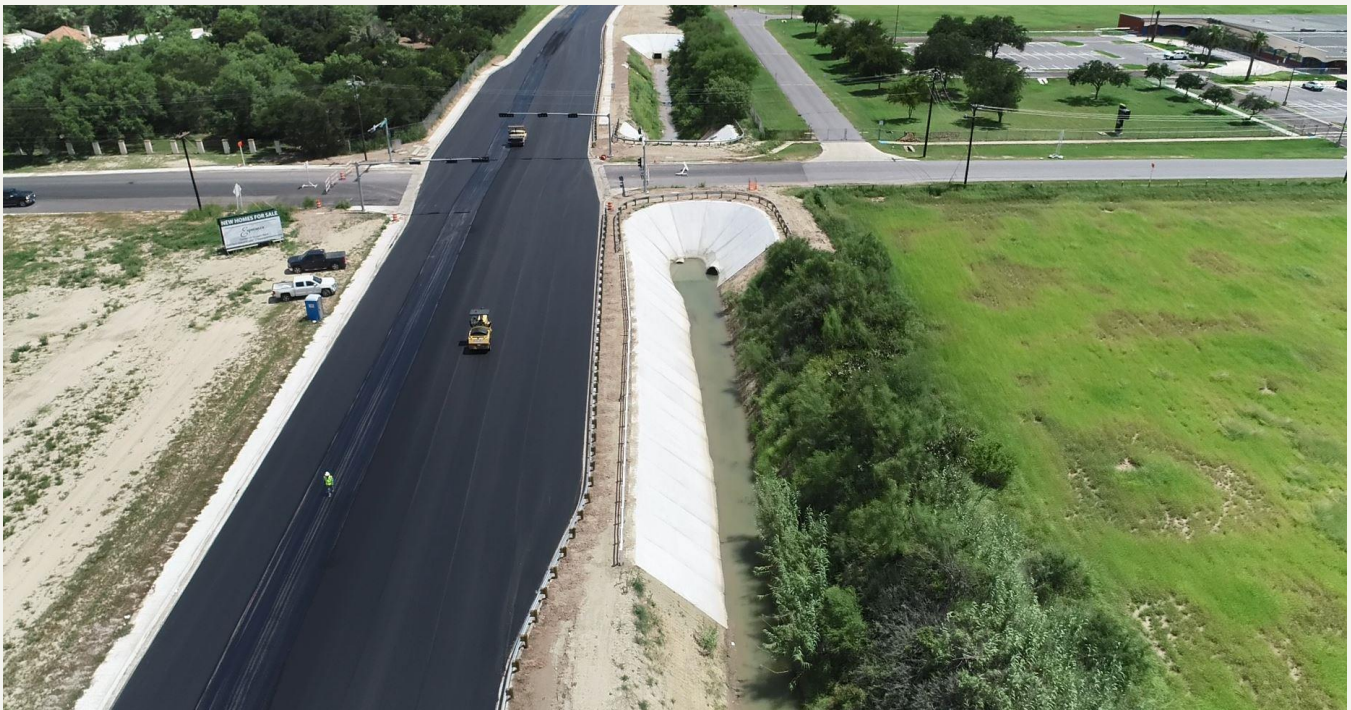
Bicentennial Blvd. Final Installation of Asphalt Surface Pavement at Freddy Gonzalez Drive Intersection.
