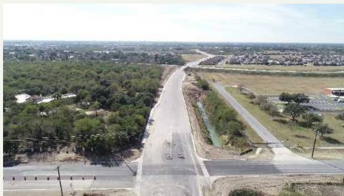
Bicentennial Blvd. Southbound Freddy Glz. to Northgate Lane
