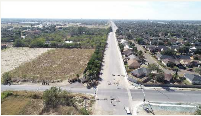
Bicentennial Blvd. Southbound Frontera Rd. to Trenton Road.
