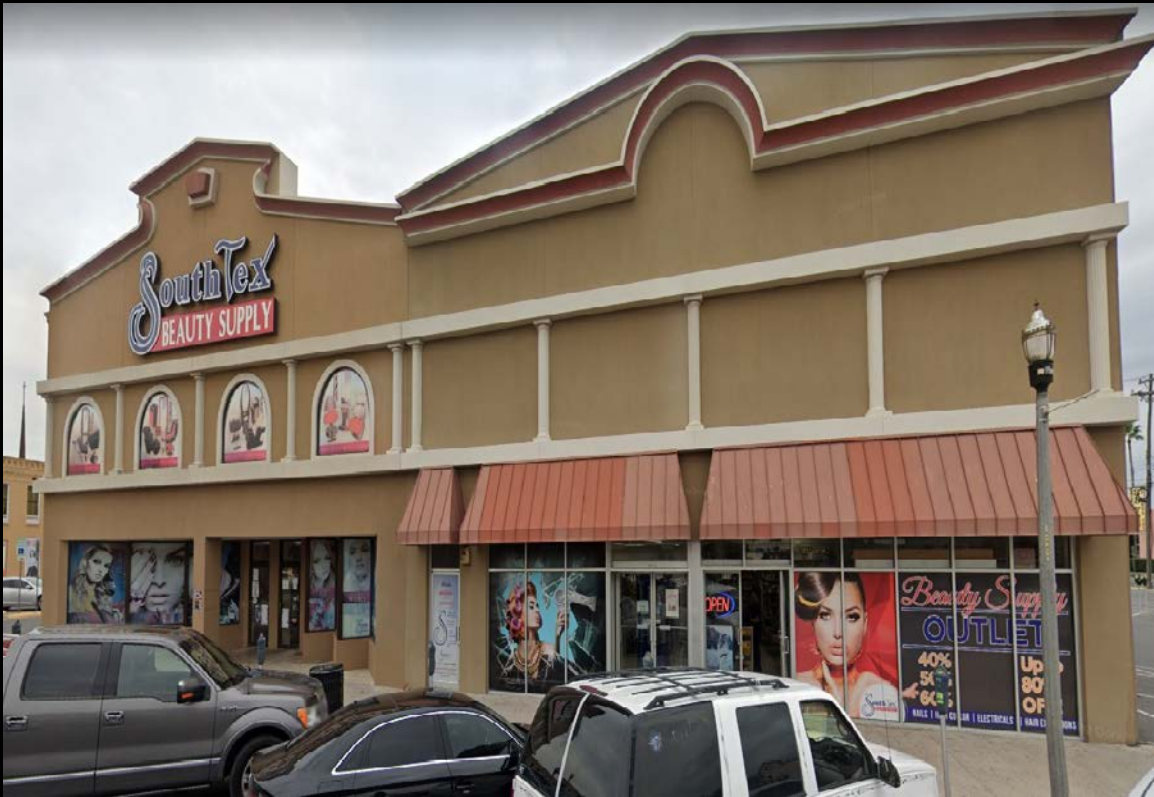
Before Front Facade
