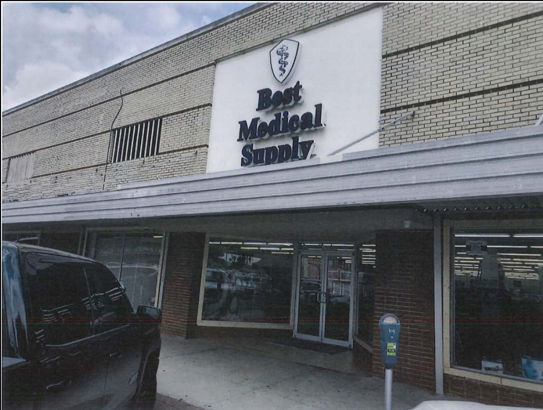
Before Front Facade
