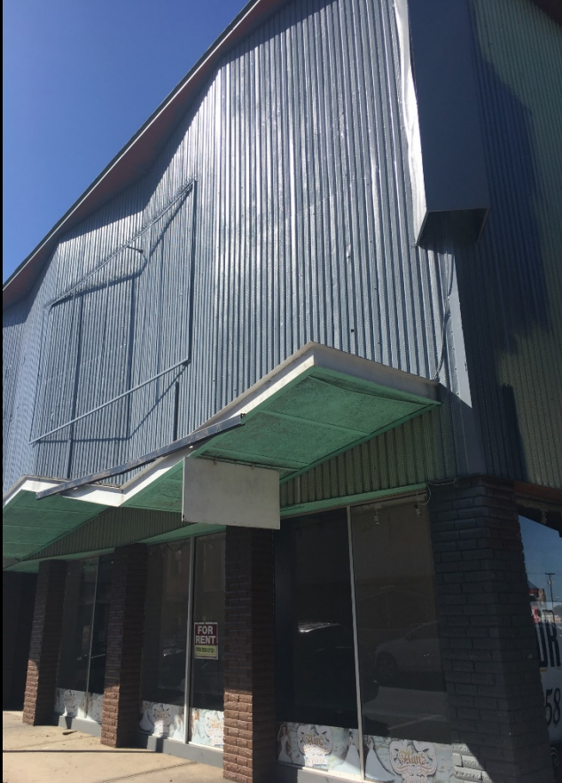
After Front Facade
