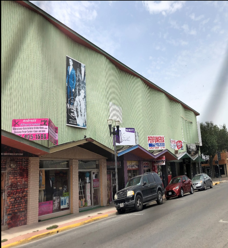
Before Front Facade
