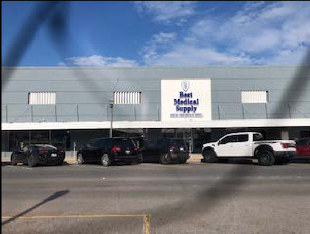
After Front Facade
