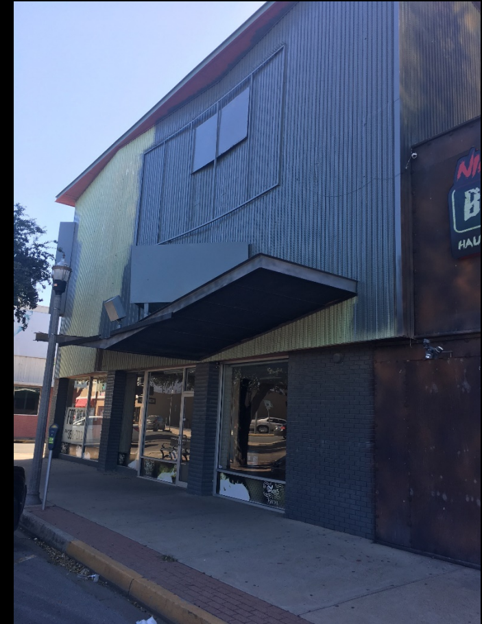
After Front Facade
