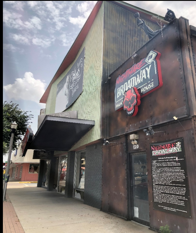
Before Front Facade
