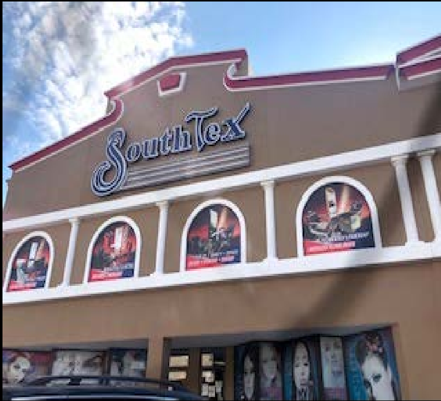
After Front Facade
