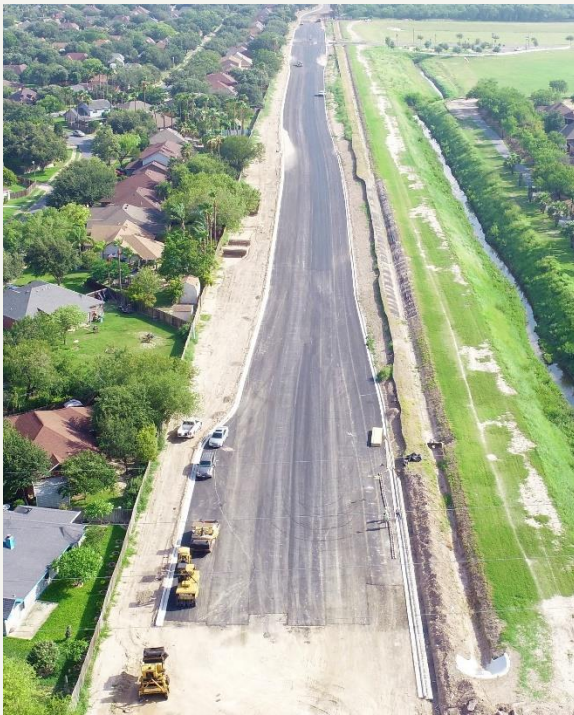
Bicentennial Blvd. Trenton Road to Auburn Ave.
