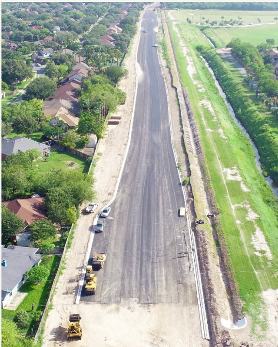
Bicentennial Blvd. Trenton Road to Auburn Ave.
